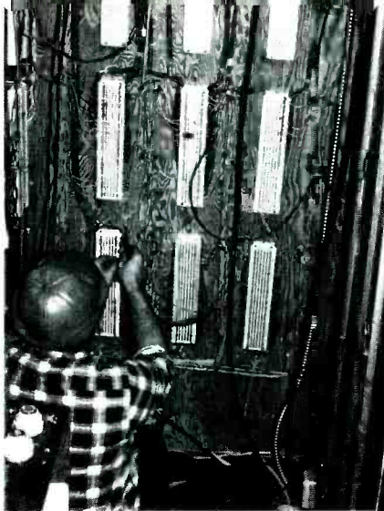
Charlie Peek, KBIA assistant chief engineer, works on wiring punch blocks of the center wire cabinet.
